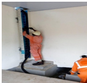
The building of Ekulama, Belame AMF Panels 2500A and Changeover panel 2000A.
